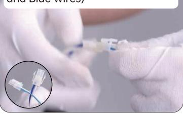
32. Use wire connecting nuts to connect the three ground wires (green) coming from the downrod, receiver and ceiling bracket
