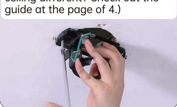
29. Place the downrod ball into the ceiling bracket. Be sure the fixation slot is locked by the bracket. If not, rotate the ball until the fixation slot is locked
