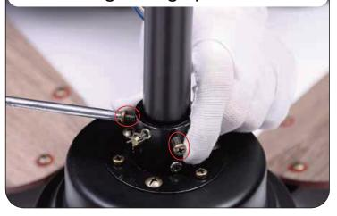
20. Remove the non-slotted canopy mounting screws, and loosen the slotted canopy mounting screws.
