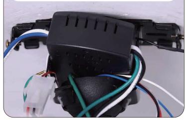
35. Lift the canopy into place and wrap keyhole slots around the screws
