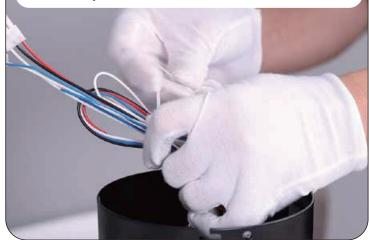
47. Connect the wire from the ceiling fan to the receiver( Red, White, and Black wires)
